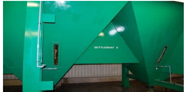
Full cone Tube Settler showing sight glasses
