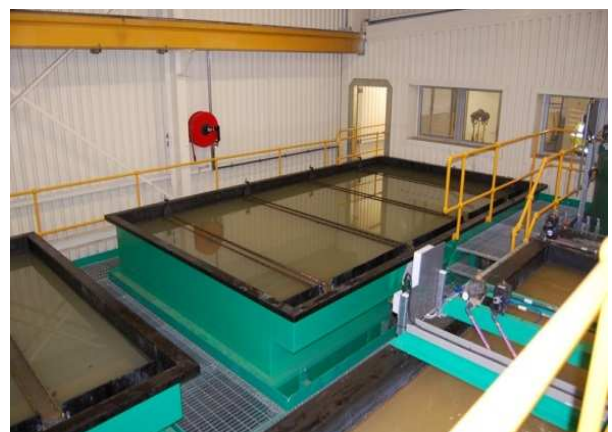
Two Tube Settlers operating in parallel
