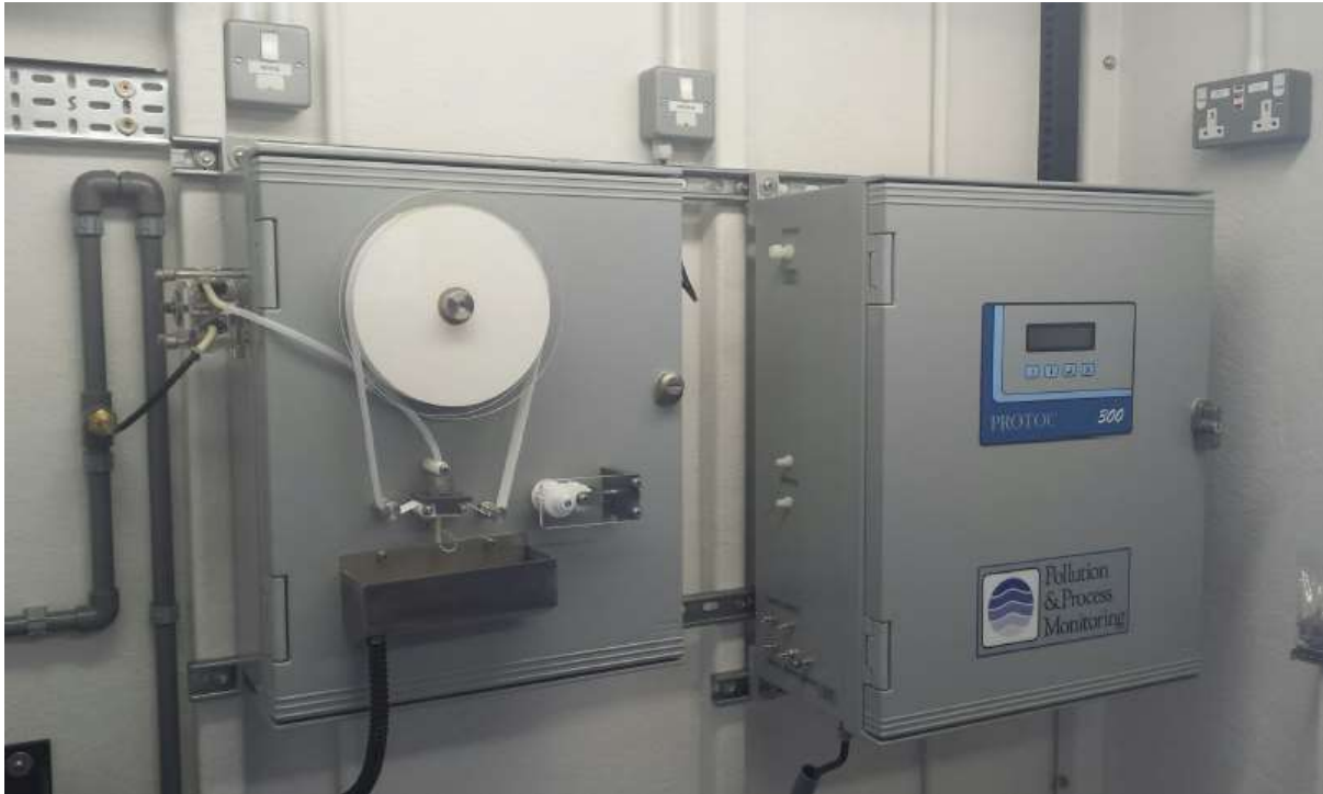
Image: Protoc 300 TOC analyser with Paper Band Filtration sample preparation system
