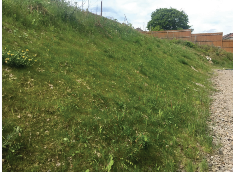
Vegetation establishing and erosion has been successfully prevented.
