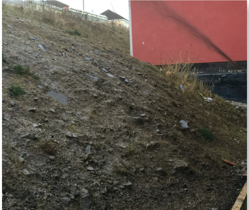
Biotic Earth applied over existing conditions where previous seeding operations failed.
