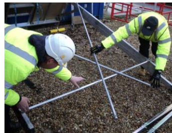
Fig 2. Secure brace.
