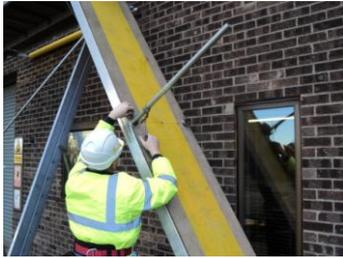
Install the Centre uprights on the Catwalk and secure with Pin and 'R' Clips. This will allow assembly of the Guardrail Set prior to access.
