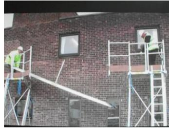
With both operatives clipped on with lanyards the Catwalk can now be raised into position. An operative must hold onto one end and guide while the second operative hoists the opposite end up until the Catwalk is Level at Platform height. The catwalk is then pulled into position with a minimum of 300mm overhang on each platform.
