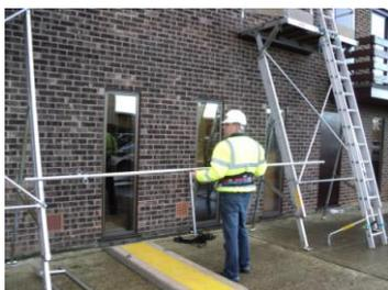
Position the two Mono-Dec Platforms 4m apart using the Guardrail or staging as a guide. **REMEMBER:** To allow a minimum of 300mm overhang of Catwalk on each of the Easi-Dec Platforms.
