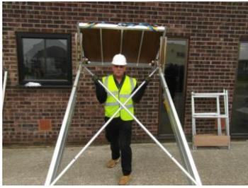
With bent Legs and a straight back, lift the Mono-Dec firstly to waist height, then using your arms to offer it to the wall and roll it up into position.
