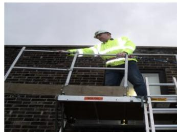
In order to prepare the Mono-Dec Platforms to receive the Catwalks, clip on with a Lanyard and remove the pin and 'R' Clips from the Internal end Guardrails and fold them outwardly. Repeat for the second Platform. This will provide access for the Catwalk to be positioned. Repeat **STEPS 1-20** for the assembly of the second Mono-Dec Platform.
