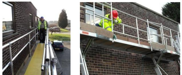
Fit the inner Guardrail the same way as in **STEP 9**. Remember to be clipped on with a lanyard at all times when fitting the Guardrails whenever possible.
