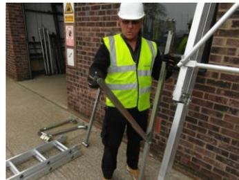
Fit the Back Legs by removing the Middle Pin first, holding onto it and lowering the brace.
