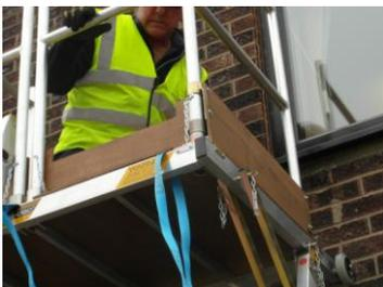
Climb onto the Platform and position the rear Uprights into the rear locating sockets on the platform for both the Left and Right handed Guardrail. Make sure all uprights have been secured with Pins provided.
