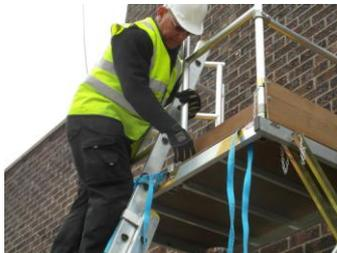
Feed one arm through the top rung of the Ladder and fit the Right Guardrail into the two front sockets and gently ease the back of the Guardrail open. **(NOTE: Always Feed one arm through the top rung as this provides a handhold when positioning the Guardrail.)**
