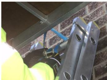
Secure the Mono-Dec Platform to a solid substrate, ensuring the wall tie is securely fixed. Consult a fixing specialist if unsure.
