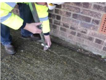
Drop the Feet to the ground and take them up to the next hole and secure with the Pin and 'R' Clip. Ideally a finger's clearance under them will ensure the Mono-Dec Platform remains in contact with the wall.
