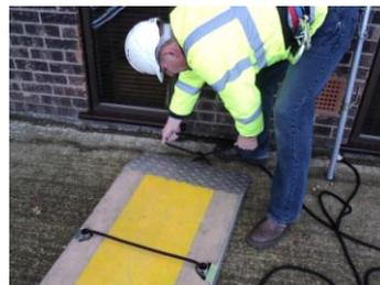
Tie a rope through the end Guardrail sockets and secure.
