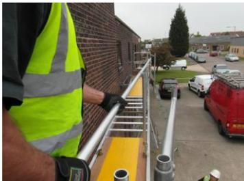
Whilst still clipped on fit the end Uprights and position the front Mid-rail and Top-rail over the Uprights from the 2m Platforms. Tighten all grub screws and secure Uprights with Pin's and 'R' Clip's.
