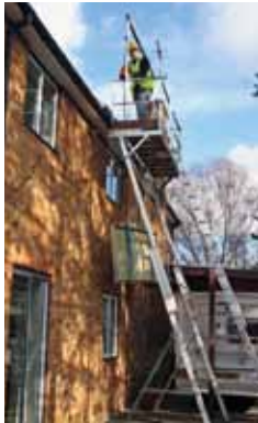
Hoisting to height
