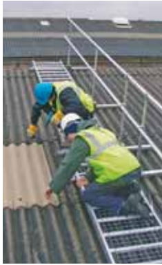
Short duration maintenance
