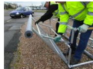
Fig 3. Lowering the panel frame
