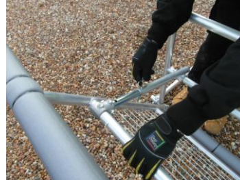
Fig 3. Lowering the panel frame
