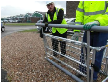
Fig 3. Lowering the panel frame
