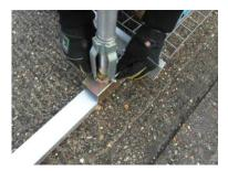
Inset the second upright in to the Batten and insert the pin and 'R' clip supplied.
