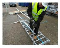
Fit the top rail into position over the uprights and tighten the grub screws.
