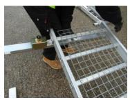
Attach the first support Batten to the Board-Walk section using the captivated pins in the hole in the stiles.
