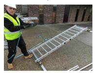
With the strap tied on securely lower the Board-Walk panel onto the roof. You would repeat these steps for further Board-Walk panels. This picture is for demonstration purposes only.
