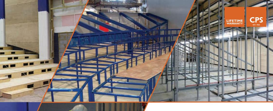
CPS offer a range of both structural steel and timber framed tiering/terracing systems. Providing an integrated seating and terracing system is often the most desired and a more cost effective alternative to cast concrete.
