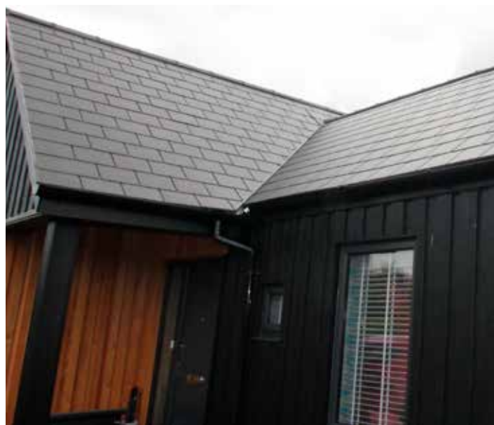
Continuously ventilated monopitch ridge
