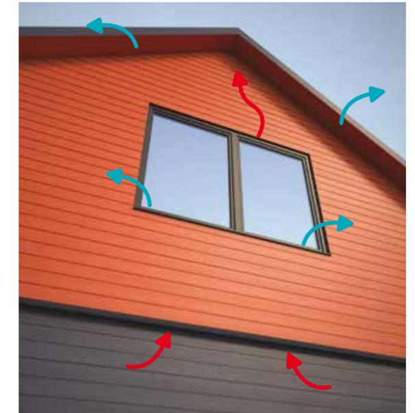
This passage must be a minimum of 10mm in the top and bottom or equal 100mm per m<sup>2</sup>. If grids or similar are used, the openings must equal 100cm<sup>2</sup> per linear meter. Cembrit offers several profiles that make it easy to create elegant solutions in the bottom and top of the cladding as well as around doors and windows.
