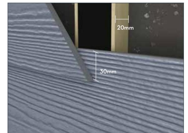
For fast, easy and accurate installation, we recommend using a Cembrit Gecko Gauge. The Geckos assist in creating the correct overlap and ensure proper location of the screw or nail. Using a Gecko Gauge set clamped to either end of the Planks, makes it possible for one man to install Cembrit Planks.
