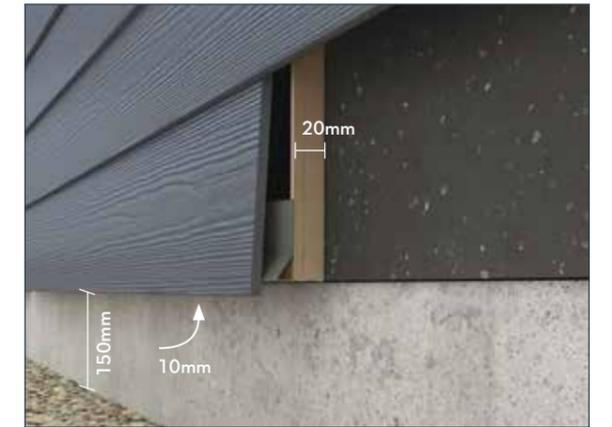
Cembrit Plank can be installed together with a Cembrit Windstopper.
