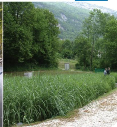
From their first application as a tertiary treatment, 'final polish', solution through secondary treatment, including nitrification, reed bed wastewater treatment systems are now widely being used for the full treatment of sewage all over the globe through the application of the **Phragmifiltre** system.
