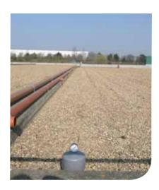
design flow of 40l/s, the wetland cells consisted of open water zones and gravel zones and were planted with *Phragmites australis*. The original system operated passively with oxygen transfer rate of  $2.4-7.7~\text{g/m}^3/\text{d}$ , removing  $4-13~\text{g/m}^3/\text{d}$  of COD. This system was unable to treat current volumes of effluent and was failing to achieve compliance.
