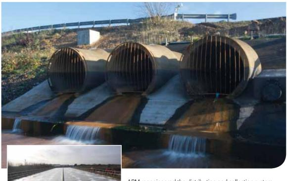
ARM reengineered the distribution and collection system and retrofitted FBA™ into the existing reed beds. The open water zones were filled with gravel and the gravel depth increased by 500mm. The upgrade works at the Mayfield Farm included the addition/modification of:
