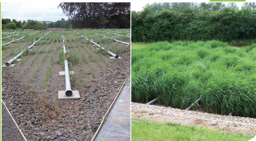
The vertical flow (VF) systems comprise a lined excavation filled with media such as sand or gravel media and unlike the horizontal flow systems, VF systems media is often graded. VF systems can have a smaller footprint than HF systems and can cope with stronger effluents. Effluent can be dosed in a variety of ways including pulse-loaded (batch), recirculating vertical flow, continuous downflow and fill-and-drain (tidal flow) wetlands. The effluent is distributed over the bed until the surface
