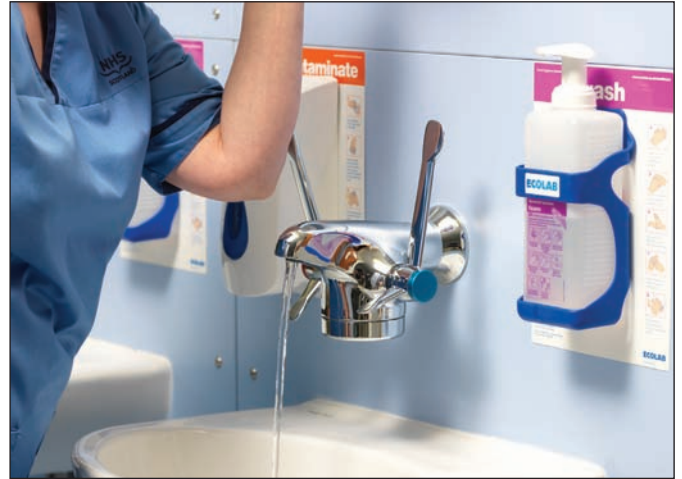
To aid hygienic handwash, the Optitherm's double lever operation allows the tap to be operated using the thumb, then turned off using the elbow or upper forearm, while the outer surface is continuous and smooth for easy cleaning.
