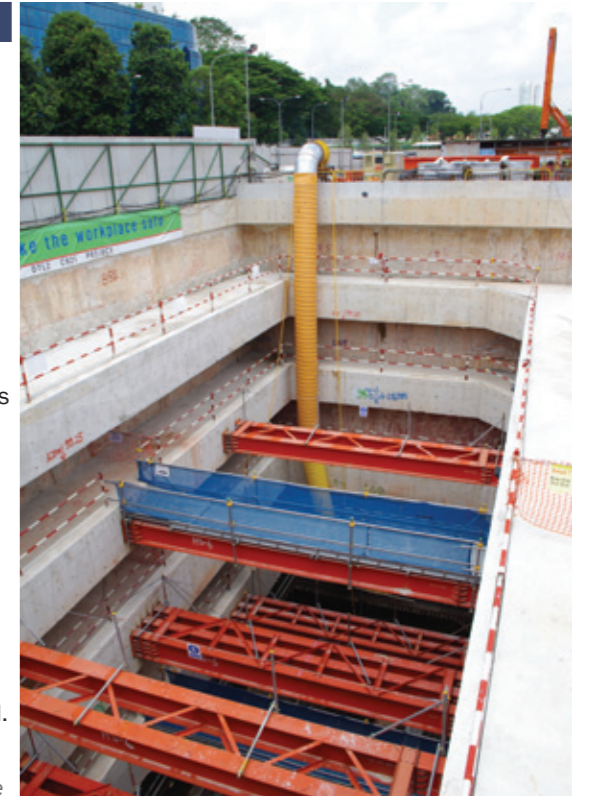
Marina Coastal Expressway (MCE) Road Tunnel, Singapore
