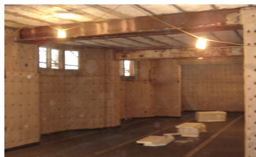
BBA approved cavity drain membrane Newton 508 Mesh in situ
