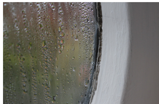
Condensation to the walls is eliminated and now only forms on the glass of the window
