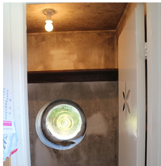
Condensation was causing unsightly damp patches on the walls
