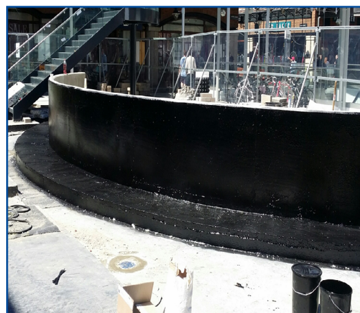
As a single-component, cold-applied membrane, Newton 109-LM was quick and easy to apply to the retaining walls and adjacent deck areas
