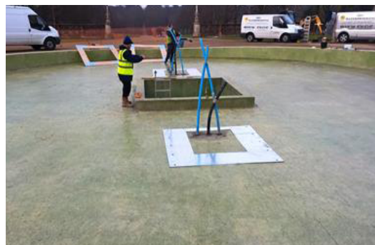
Application of Newton 903-Primer to the 10m diameter fountain base
