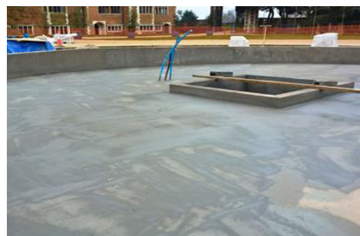
Newton 103-S was spray applied to the base and the upstands
