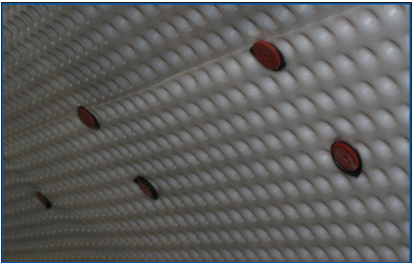
The Newton System 508 Cavity Drain Membrane applied to upgrade the existing tunnels in the London Underground station using Newton Nuseal Plugs and Newton Waterseal Rope
