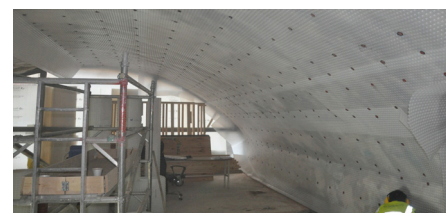
Application of BBA certified Newton 508 Cavity Drain Membrane to the vaulted areas
