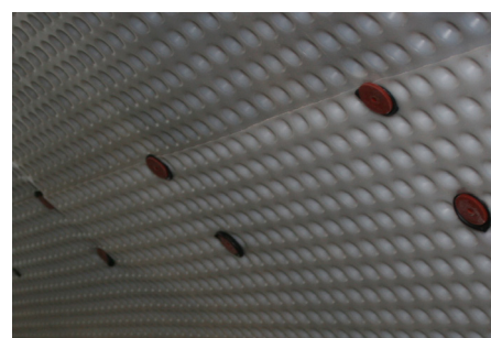
WaterSeal Rope was wrapped around the neck of the plugs to form a waterproof seal
