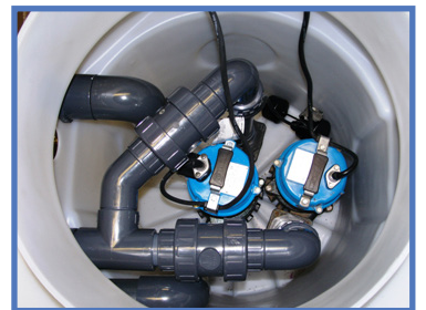
View of 2 x NP400 pumps in a Titan-Pro White Sump chamber
