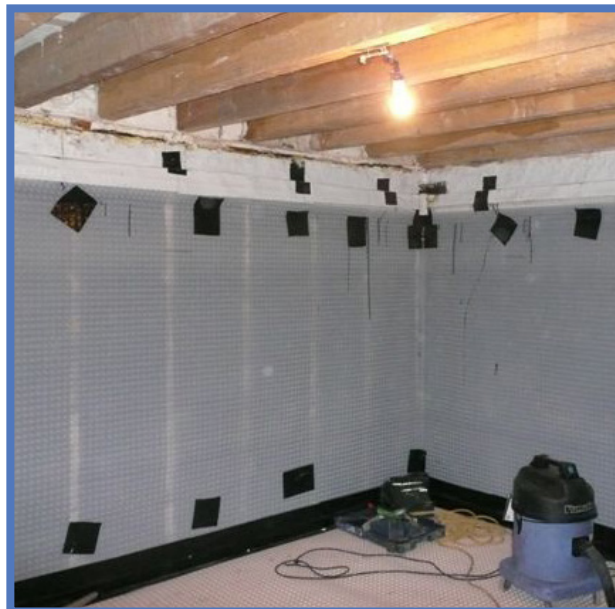
Newton PAC-500 System installed to a house in Derbyshire with very high levels of Radon gas
