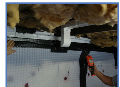
Air inlet manifold installed and shown being integrity tested
