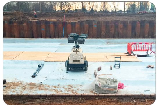
Heavy objects can be placed on top of HydroBond
