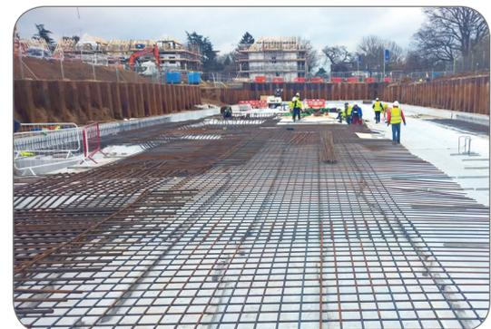
Reinforcement steel can be placed on top of the HydroBond ready for the concrete to be placed
