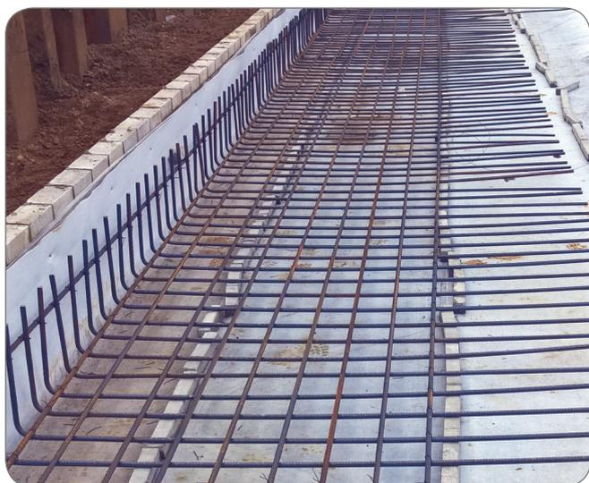
*For good practice, concrete spacers are placed on top of the 70mm lap to reinforced this joint*
