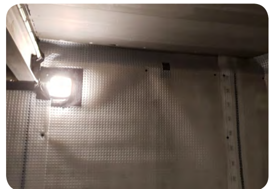
4. The CDM installation also required some high quality detailing from the Wise specialist installers
