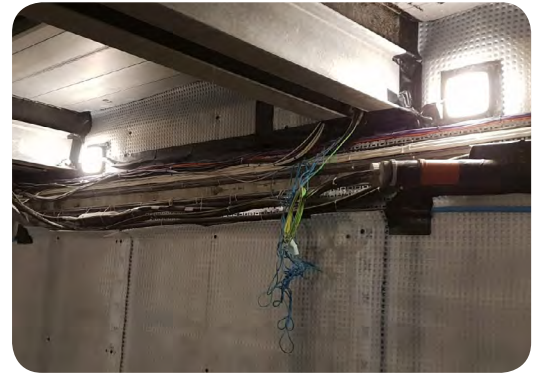
3. The CDM System also had to accommodate numerous existing lights and cables/services
