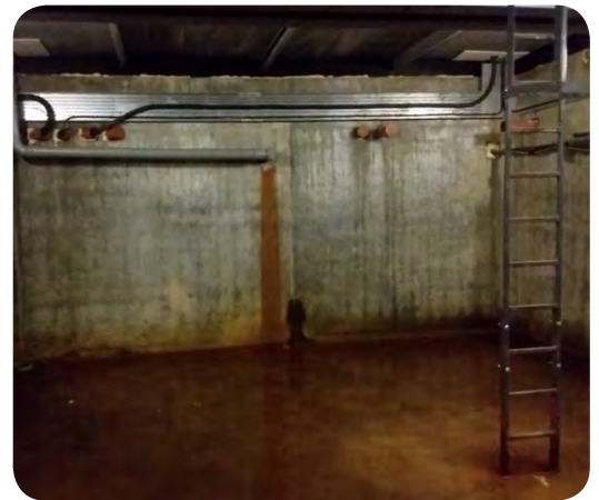
1. The basement of the Air Traffic Control tower had 2 inches of water and water ingressing through the walls
