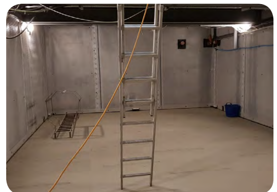
5. With the CDM system in place and a new floor down, the basement has been transformed
