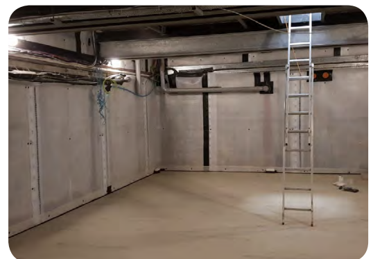
6. The waterproofed basement is now completely dry and ready for use by the client
