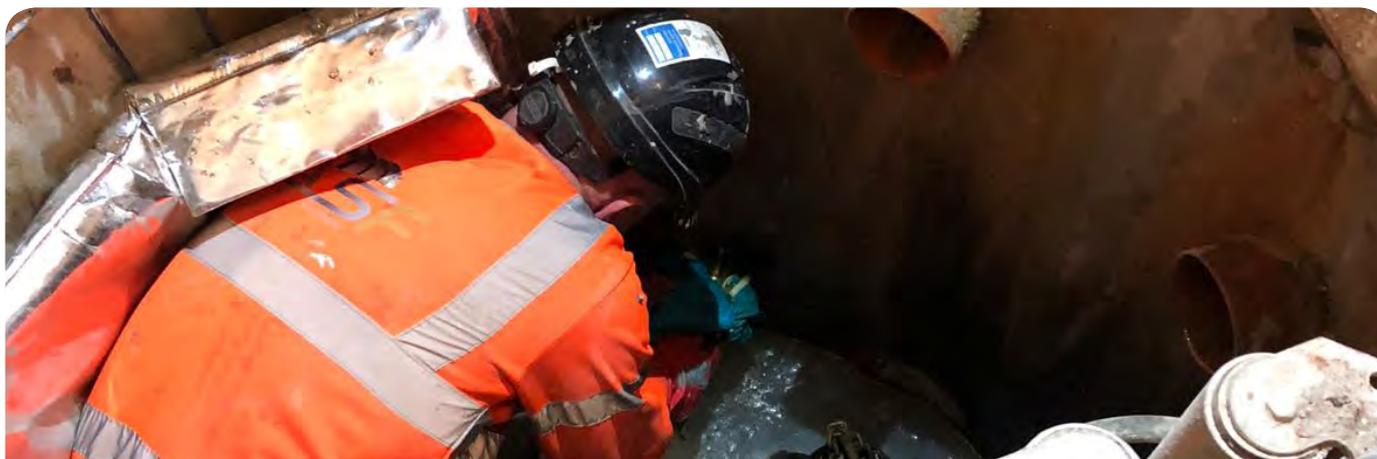
Polyurethane Injection Leak Sealing in a Basement Tank, London
