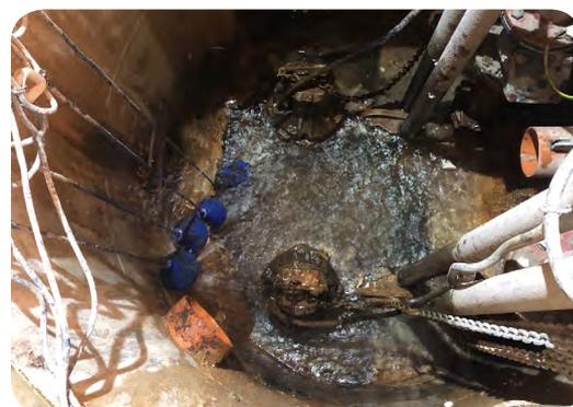
1. The cracked tank in the basement was allowing the ingress of large volumes of groundwater
