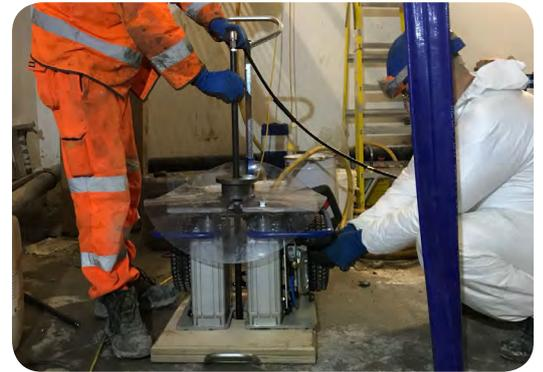
4. Once injected into the substrate, the 320-FP reacted quickly with the ground water to provide a seal
