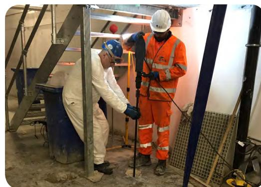
2. ASF Waterproofing first drove packers down through the slab to a depth of 2.5m around the tank
