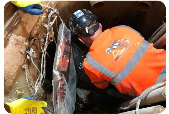
5. With the flow of water stemmed, ASF Waterproofing could now get inside the tank to inject Newton 322-SP
