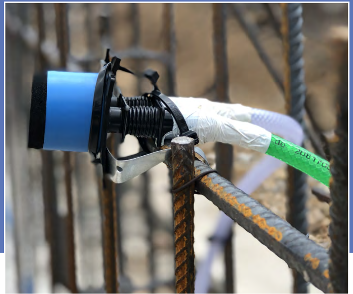
Injection ports were installed every 10-metres
