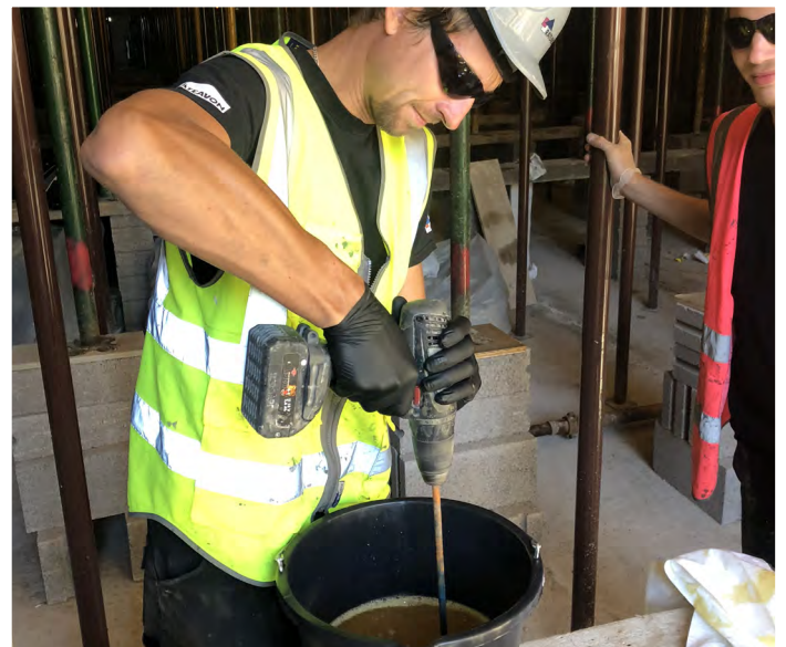
Newton 322-SP is quickly and easily mixed on-site
