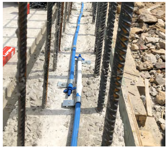
Injection Hose is installed in 10-metre lengths
