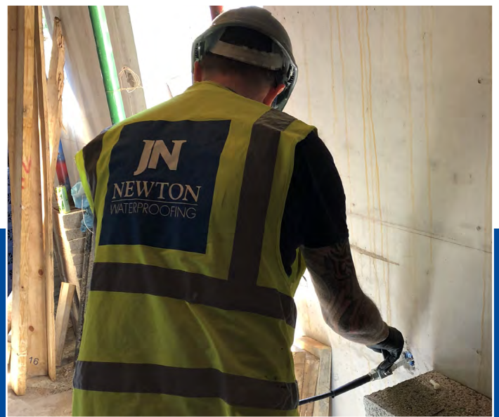
The one-shot resin fills any voids and cracks within the construction joint
