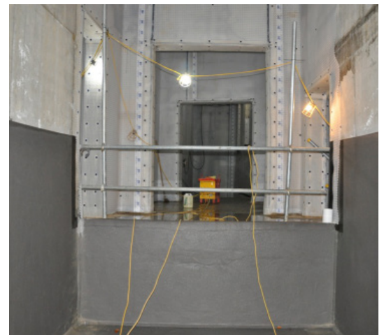
Newton 107F applied to the internal lift pit.
