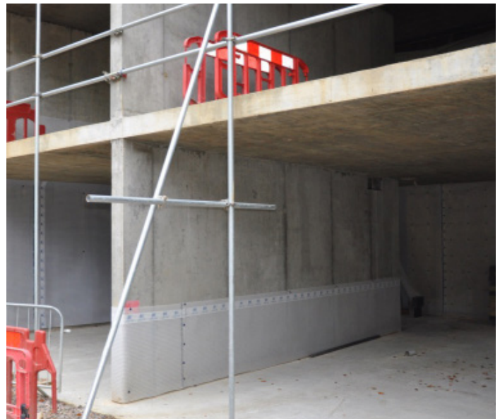
The Newton CDM System is failsafe and fully maintainable.
