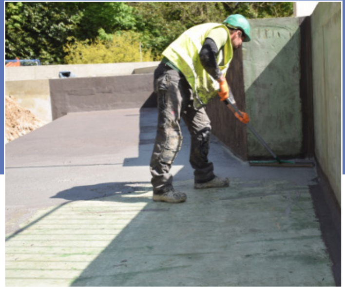
A cementitious coating was applied to the external flat roof.
