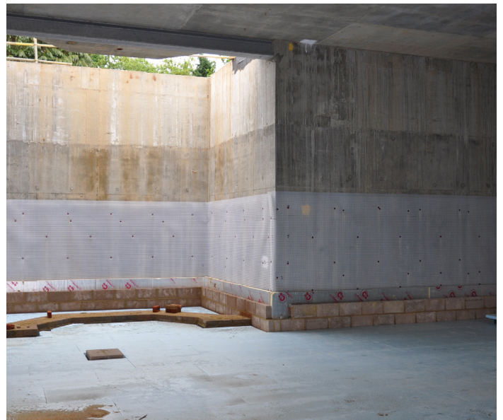
The new below-ground concrete structure was extensive.
