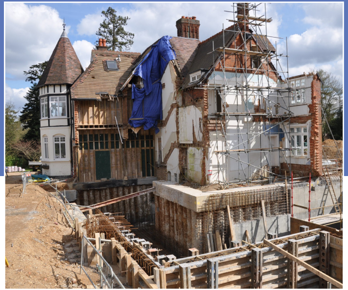
A large extension and basement was added to the existing structure.
