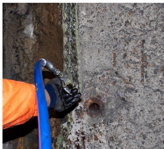
Water was leaking in from near the roof of the tunnel.
