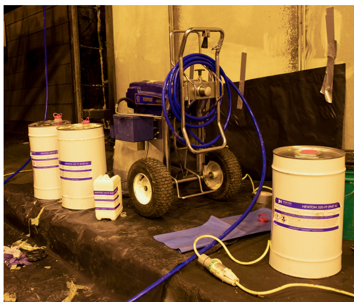
A Graco machine was used to inject the specialist resin.
