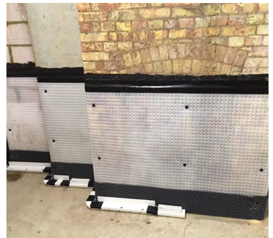
The project involved new and existing structures.
