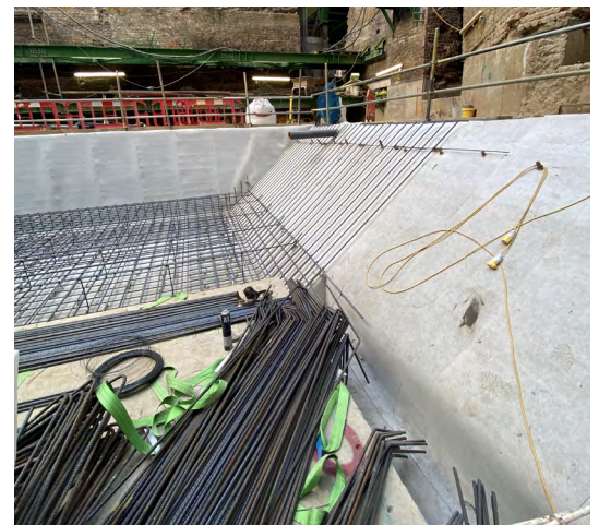
403 HydroBond applied to the new attenuation tank
