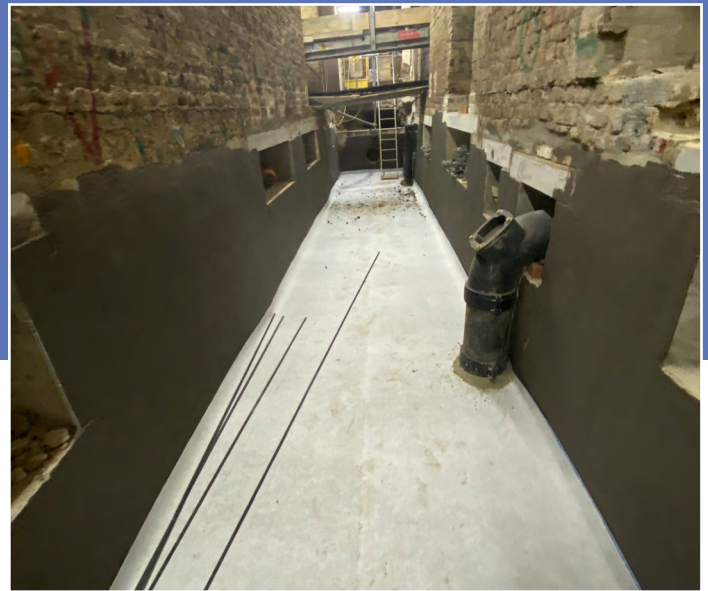
403 HydroBond and 107F used in conjunction in Building 2
