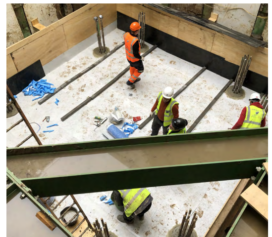
Installing HydroBond prior to a concrete slab install
