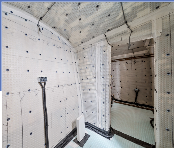
Newton 508 Mesh was installed throughout the Listed basement
