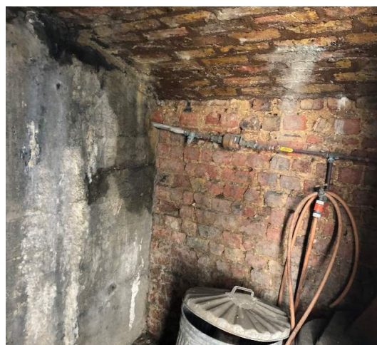
The existing basement vaults were extremely damp.
