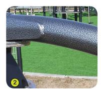
2- The 60mm diameter tube is made of lacquered steel.
