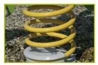
5- The springs are made from Grade 35SCD6 steel, shot blasted, stress relieved, zinc coated and finished with two coats of epoxy polyester powder.
