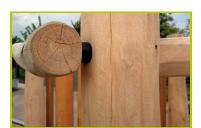
1- The different posts (60 to 80mm / 100 to 120mm / 120 to 140mm) are made from sap free robinia. The robinia is sanded and has had its bark removed. Robinia is naturally rot proof and does not require any additional chemical protection; it is equally extremely resistant to attacks from external sources (insects, fungi, climatic variations), guaranteeing the long term durability of the playground equipment.
