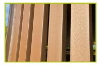
**5- The slatted fences** are made of composite wood (slats of 70 x 30 mm), which is a chip and split resistant waterproof material with UV protection.
