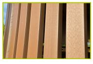
**5- The slatted fences** are made of composite wood (slats of 70 x 30 mm), which is a chip and split resistant waterproof material with UV protection.
