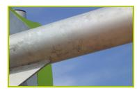
1- The horizontal beam is manufactured from 89mm diameter galvanised steel.
