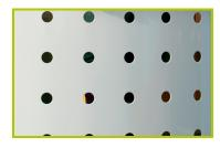
7- The balcony is made of 3mm perforated aluminium sheet, coated with polyester epoxy lacquer.
