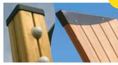
Laminated wood is made up of layers of solid wood (often Fir or Scots pine) glued together. It is a very strong material and ideal for posts that have to carry larger loads.
