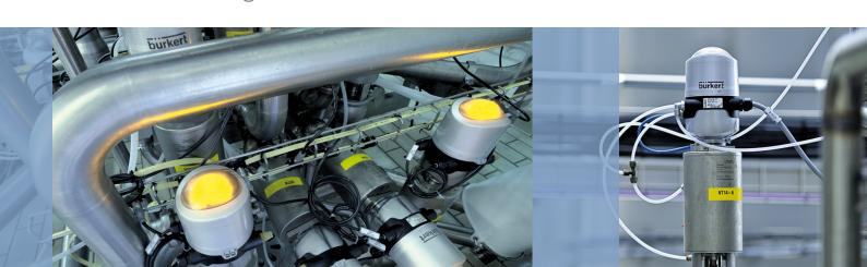
its protection rating and its resistance to chemical cleaning products. In the context of decentralised automation concepts with fieldbus communication protocols, the control head executes all pneumatic commands, position feedback functions and diagnostics. Depending on the process valve, it can control up to three pneumatic chambers separately.
