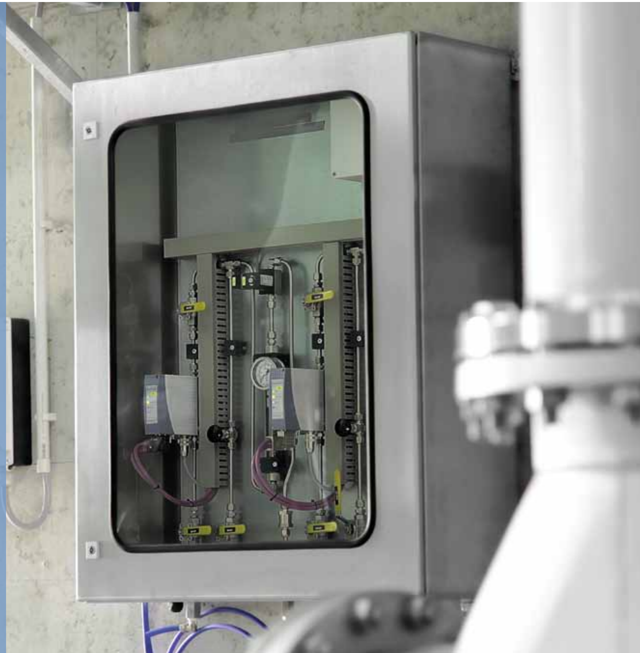
Oxidator box from Bürkert: Two-channel system in Everswinkel Municipal Utilities Waterworks
