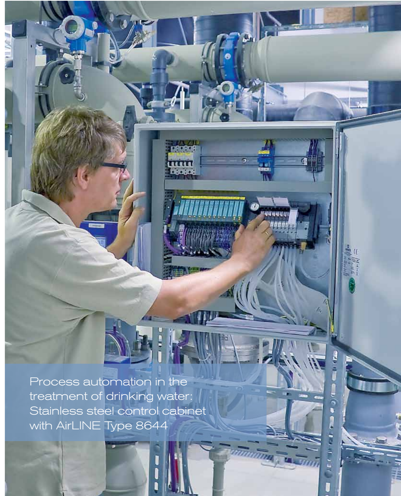
AirLINE automation system Type 8644 in water treatment
