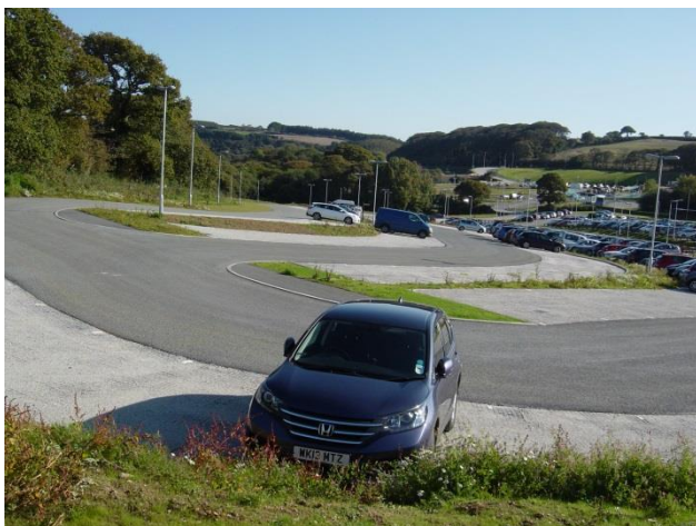
Gravel filled parking bays
