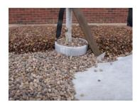
Alternatively, funnel the aggregate at the base of the tree trunk to a depth of 10–15mm below the final expected finished level. This will provide a weaker bond to allow the bond to break as the tree grows.
