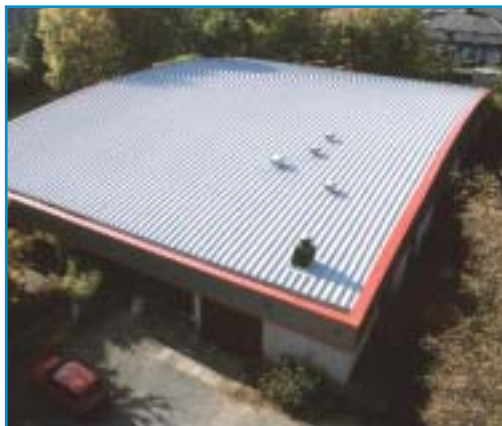
Ashjack Propped Rafter System overlaid with an Ashzip standing seam roofing system
