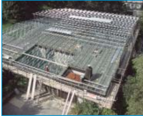
Ashjack propped rafter system during construction
