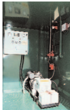
Auto-Generator for Radio Equipment
