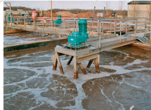
4 HYPER-CLASSIC ® Mixing & Aeration Systems in an industrial wwhp in Belgium (Food Industry)
