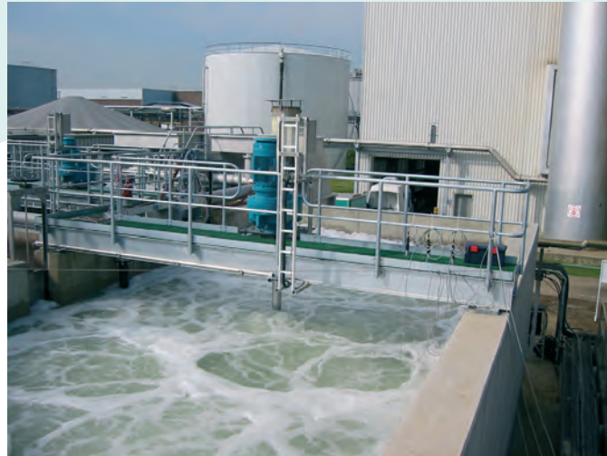
1 out of 9 HYPER-CLASSIC® -Mixer/Aerators in an industrial wtp in Belgium (Pulp & Paper Industry)
