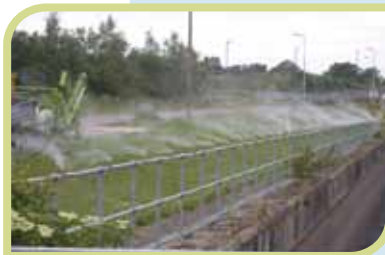
Sewage storm tank perimeter treatment
