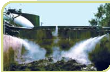
Limed sewage sludge storage bay
