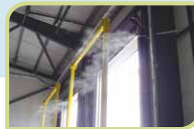
Doorway coverage at a waste transfer facility
